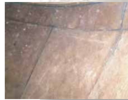
Internal armouring of a vertical crusher
